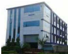
Tecnik Fluid Controls Pvt. Ltd. Mumbai, India
